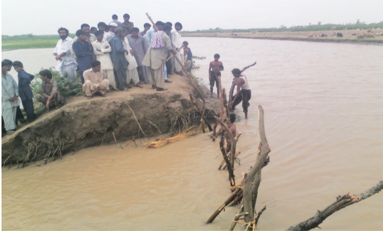
Heavy rainfalls in single months of July 2016 and August 2016, which coincides with the monsoon season.
